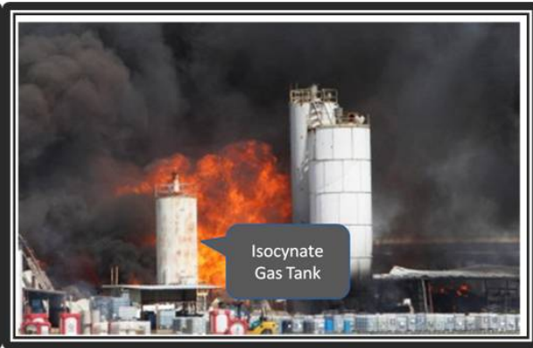
FIGURE 2 Picture showing the back of the factory and the gas tank
